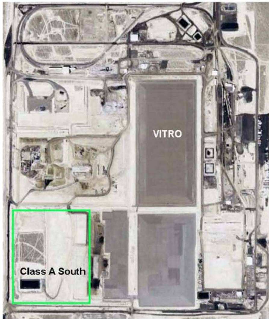
Figure 2. Disposal and Treatment Facilities operated by EnergySolutions.
